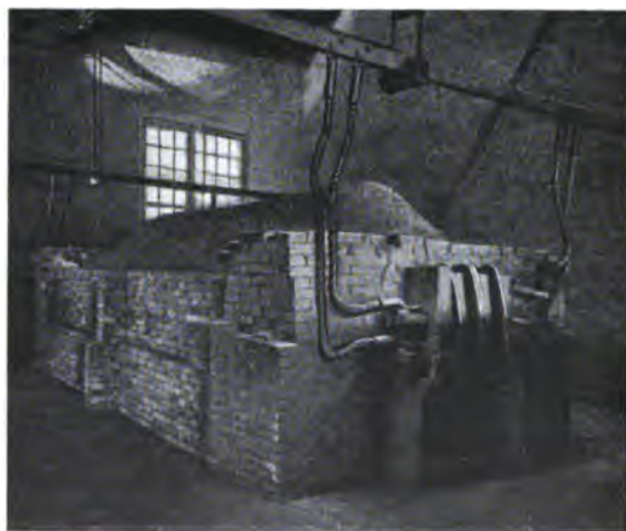
FIG. 100.—Electric Furnace for Manufacture of Carborundum.
